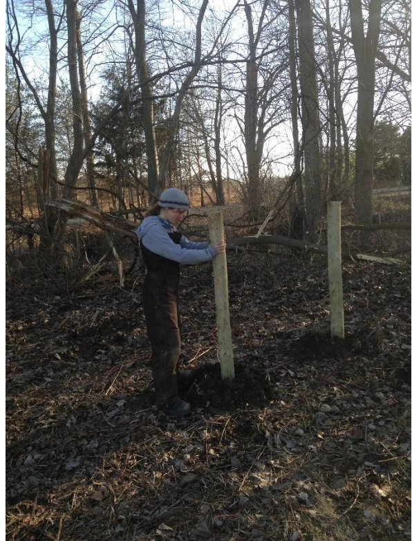
Me setting fence posts.
